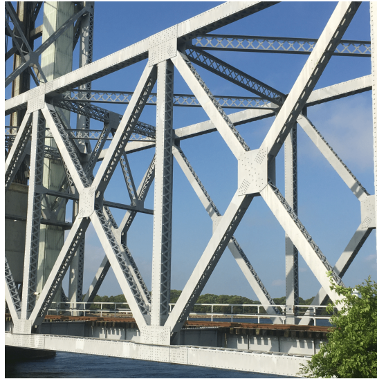
Figure 6.3.1 Truss with riveted gusset plates.
