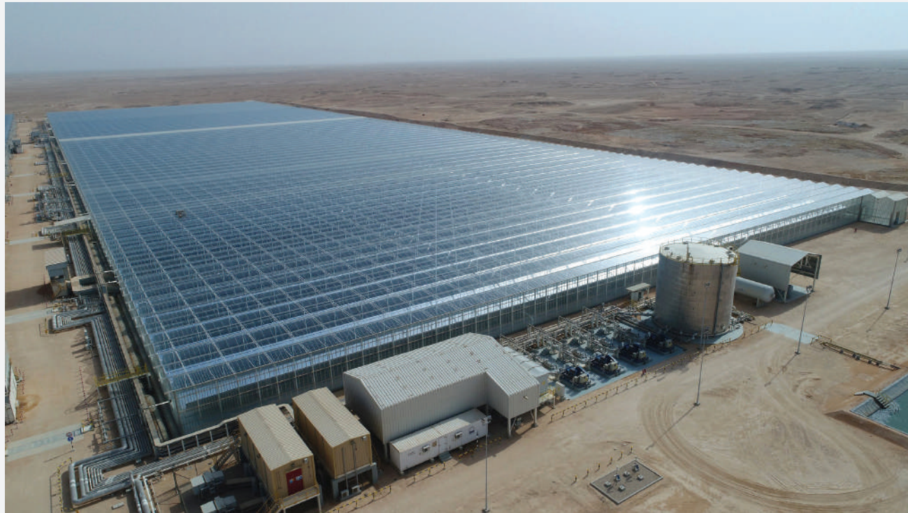
Oman's geographical location makes it ideally suited for large-scale solar power generation
