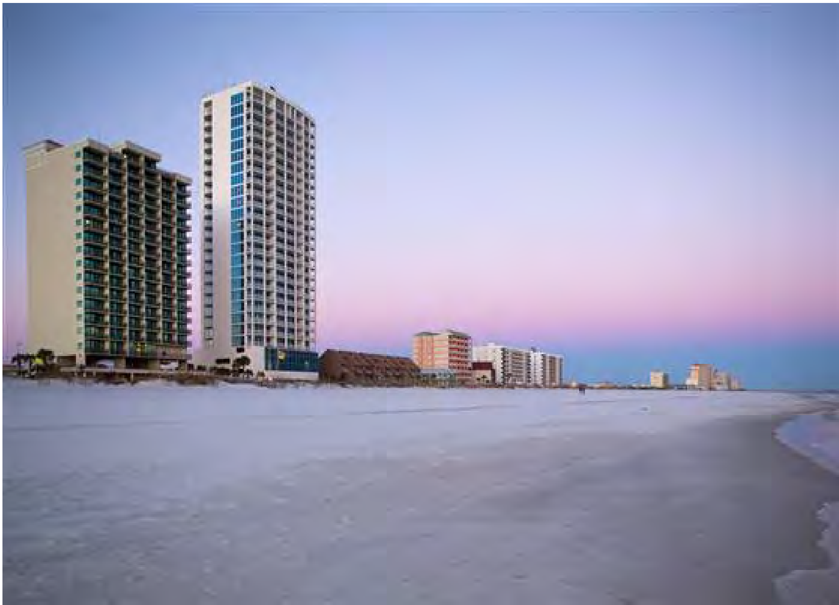
The Island Tower condominium building, right, and the Phoenix All Suites Hotel, left, rise above the beach in Gulf Shores. FEMA remapped both into lower-risk flood zones. (Photo by John Brecher / NBC News.)
