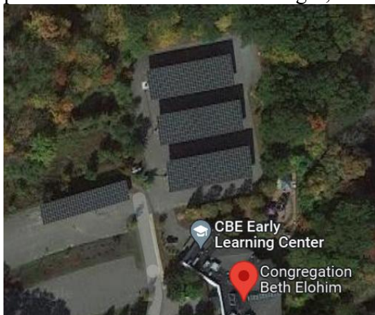
A 302 kw ground mount parking canopy solar installation at Congregation Beth Elohim, Acton MA
