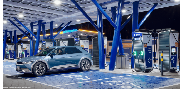
Fig. 1: Europe’s largest high-power charging hub with 26 CCS charging stations that allow a total of 52 vehicles to be charged concurrently [22].
