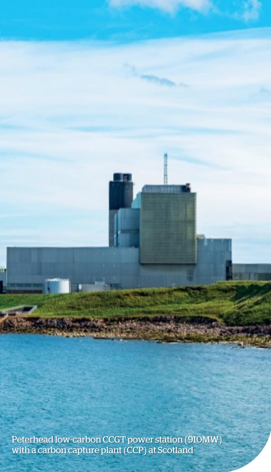
Peterhead low-carbon CCGT power station (910MW) with a carbon capture plant (CCP) at Scotland
