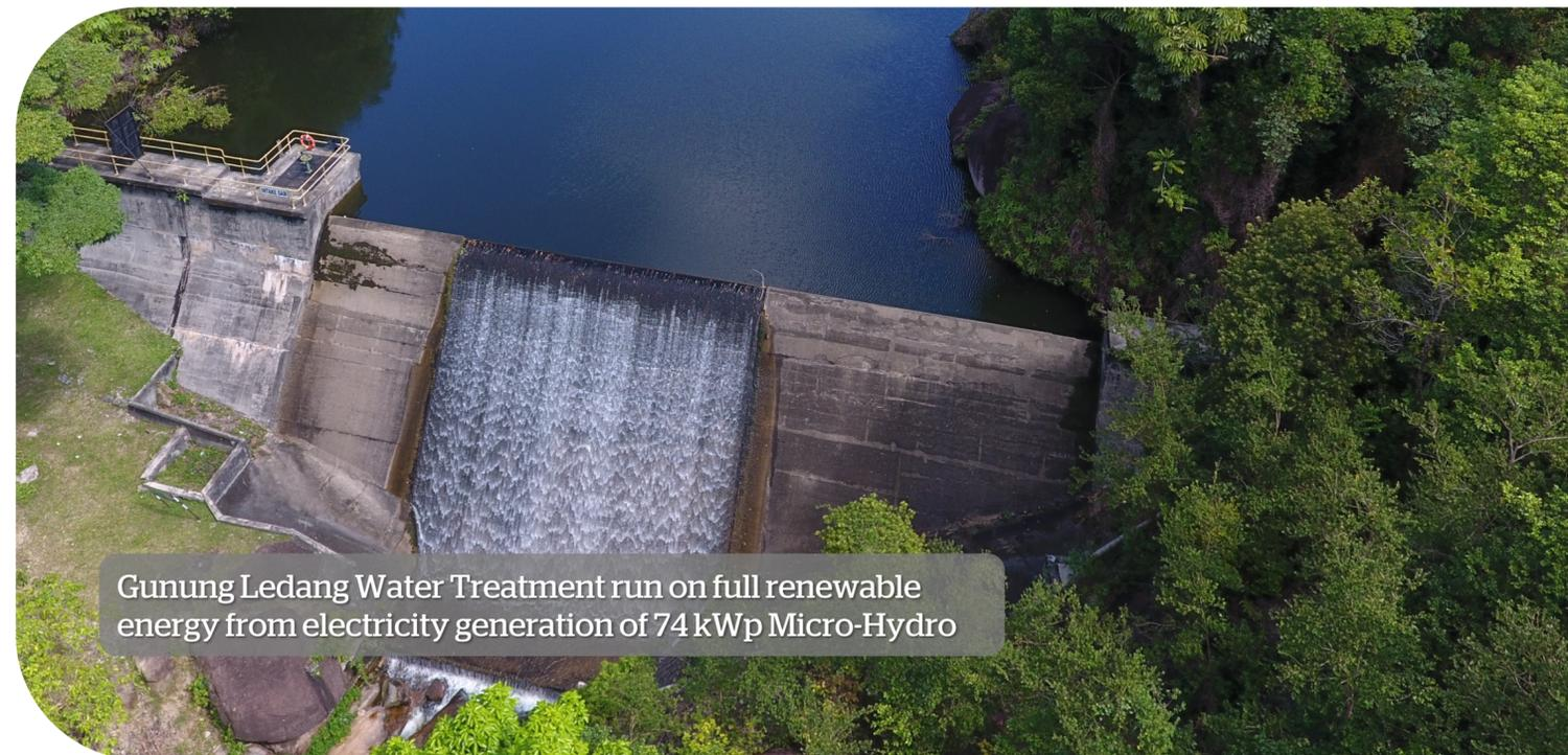
Gunung Ledang Water Treatment run on full renewable energy from electricity generation of 74 kWp Micro-Hydro
