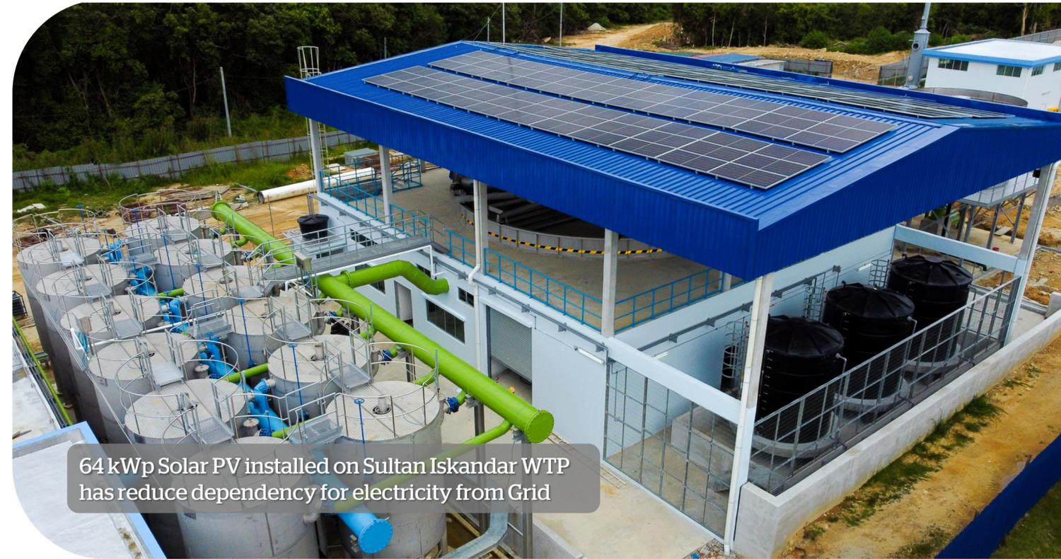
64 kWp Solar PV installed on Sultan Iskandar WTP has reduce dependency for electricity from Grid
