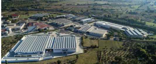
CEIA S.p.A. Headquarters, Vicomaggio, Arezzo
