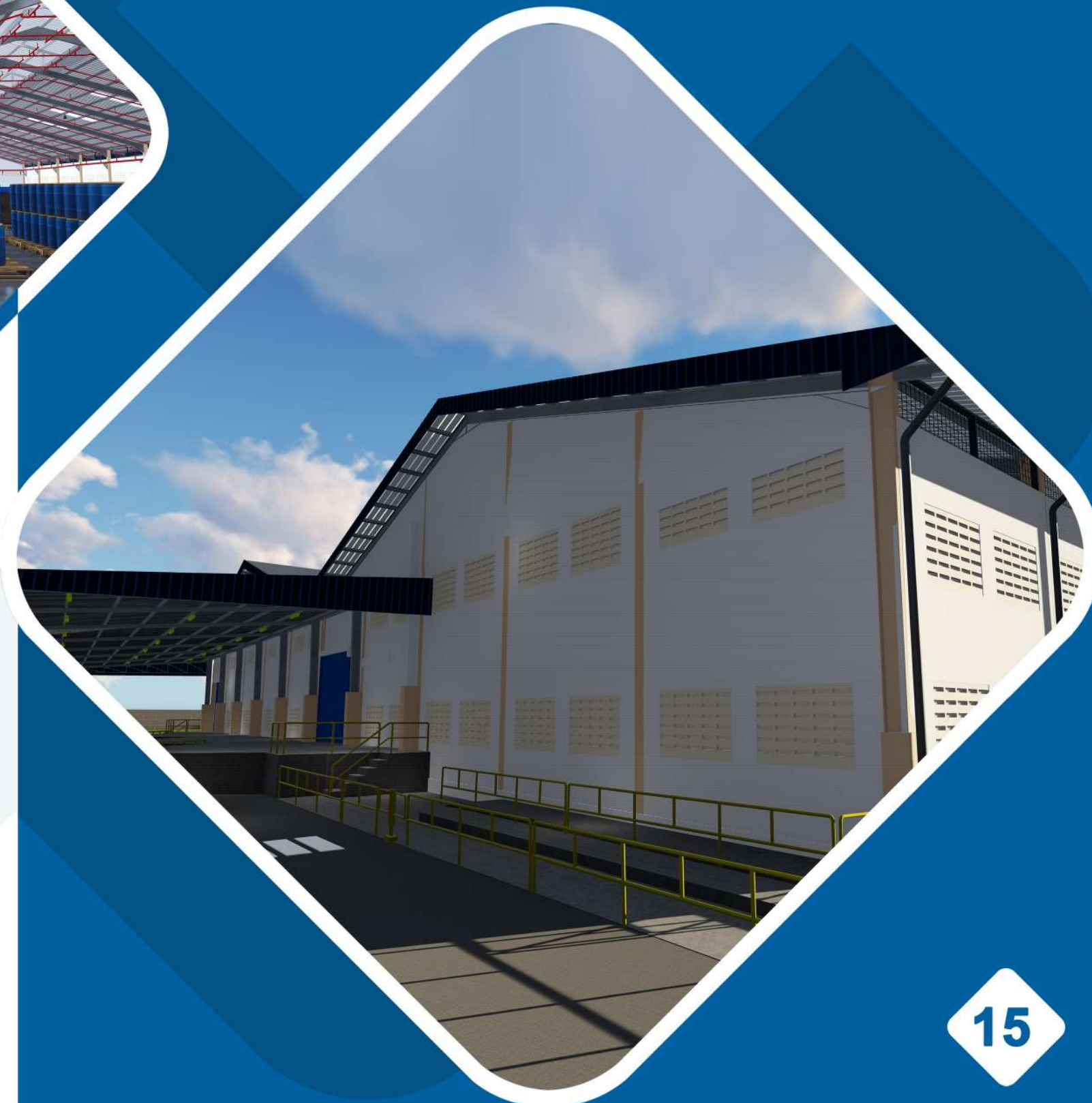
3D As Built Survey for Heinz-ABC Processing Plant
