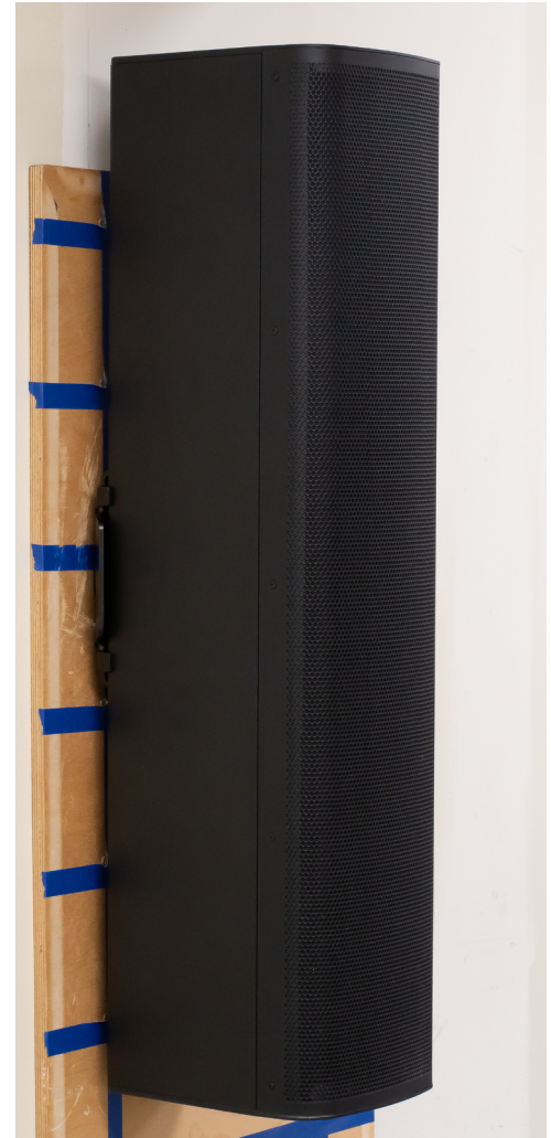
Installed flush mount bracket
