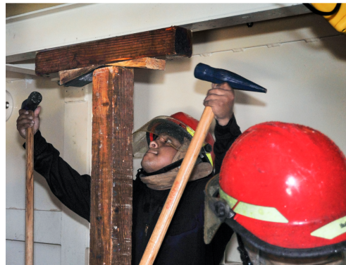
(b) High friction wedges are used to secure shoring timbers.
