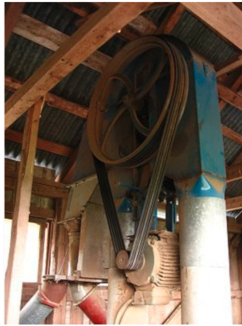
(b) Power transmission pulleys.
