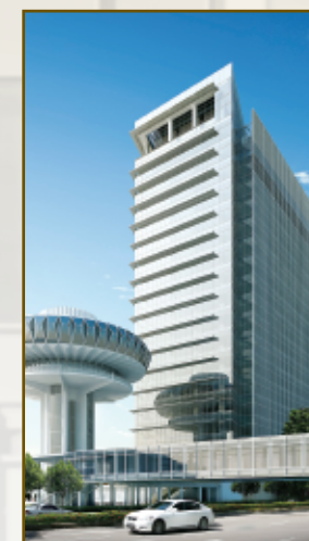
50 COLLYER QUAY (INCLUDING CHANGE ALLEY AERIAL PLAZA) COMMERCIAL
