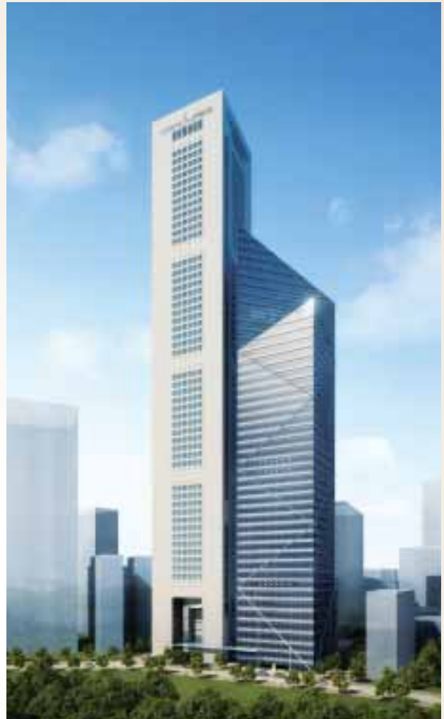
Exterior, One Raffles Place
