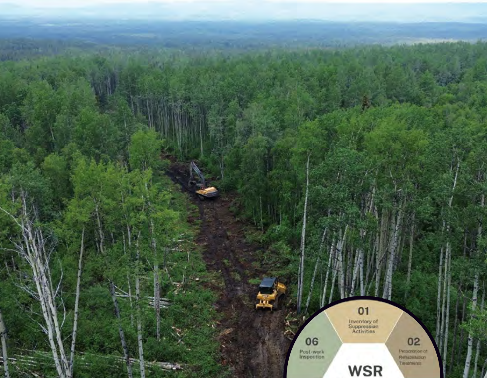
Dozer and excavator building machine guard (fireguard). Location: Pink Mountain, 2025. Photo credit: Kyle Miller, RFT.
