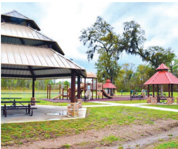
Rathborne Park sits at 702 Lakewood Drive in Luling. The parish put up barricades around the playground in early May and it will remain closed until the equipment is repaired.
