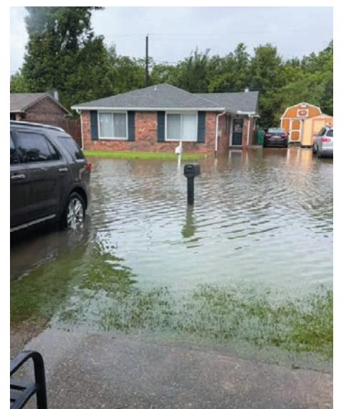
Street flooding during Tropical Storm Arthur.
