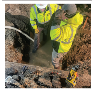
IRWA provides assistance in an excavation to locate and repair a leak in the water distribution system of the City of Glens Ferry.
