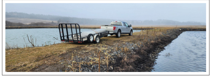
Conducting a sludge judge sampling at the lagoons of Princeton-Hampton Sewer District.
