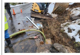
IRWA provides support during an excavation in Benewah County.
