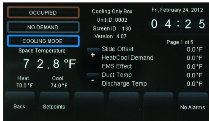
Figure 40: VAV/Zone Controller Status Screen
