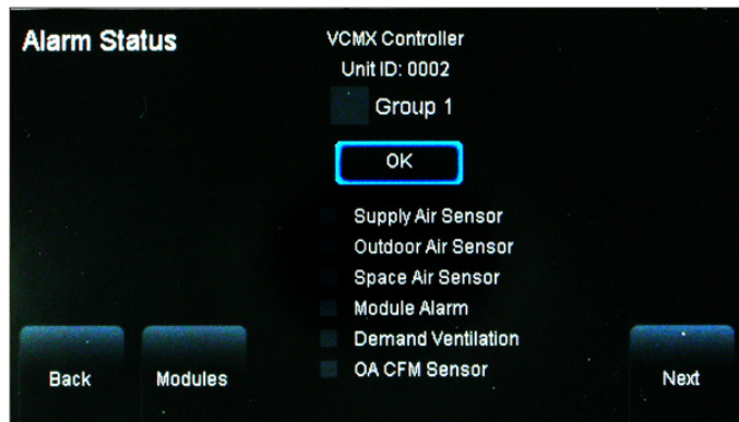
Figure 21: VCM-X Controller Alarm Status Screen
