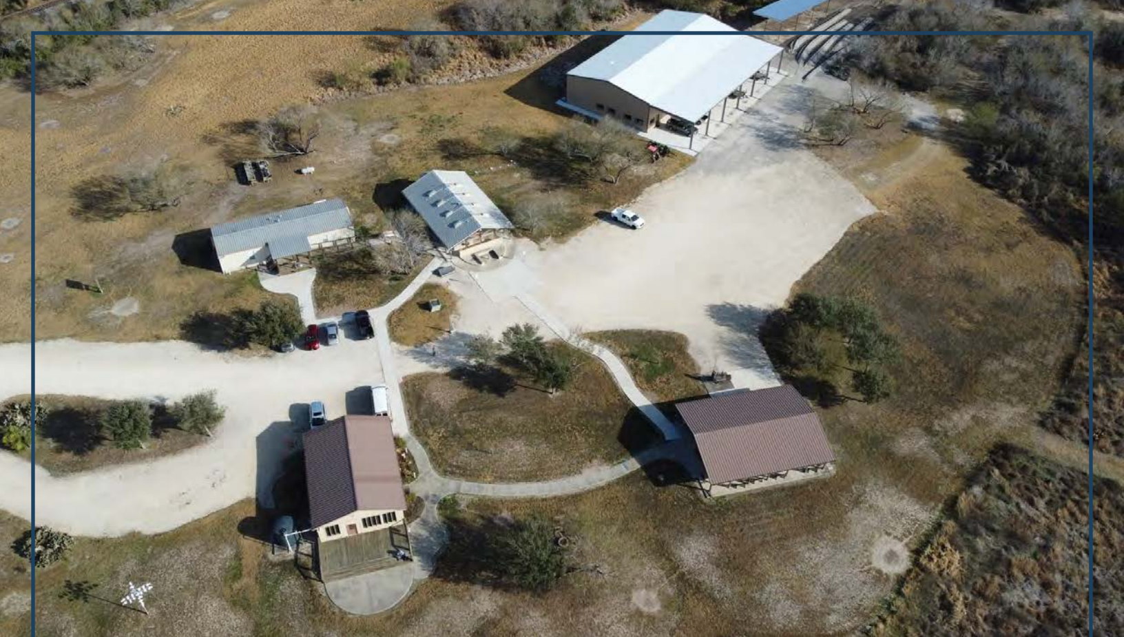
Aerial view of CBBEP's infrastructure at the Nueces Delta Preserve, including the newly constructed Land Conservation Program Building.
