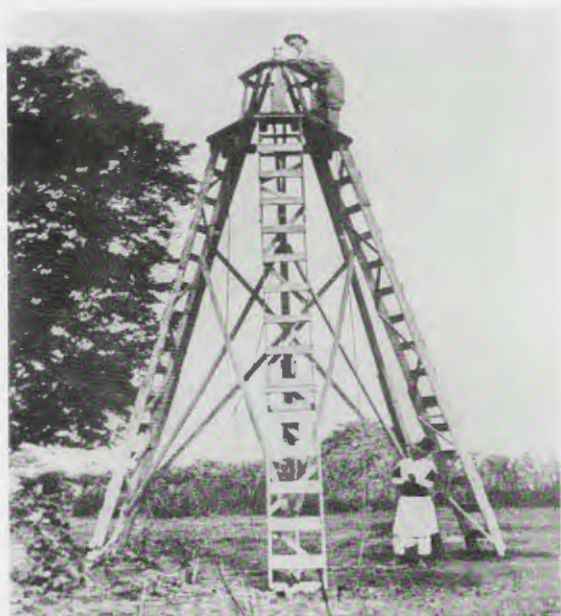
Fig. 19 (above). Trellis with dismantle platform for rising up to tree level to carry out topographical surveys.
