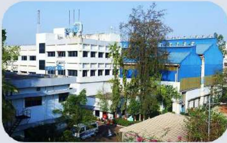
Dedicated spares manufacturing plant
