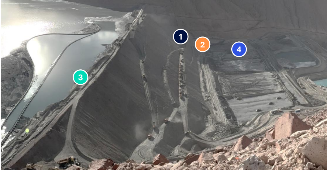
November 2025 – QB Site Visit
